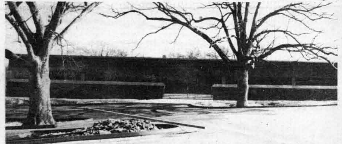
GENERAL SERVICES BUILDING: Finishing touches now being done, the General Services Building will be completed By April. UMSL Police and personnel will be housed there. [Photo by Romondo Davis]
